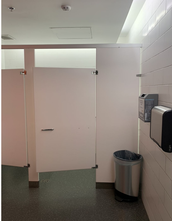
View of accessible washroom door
